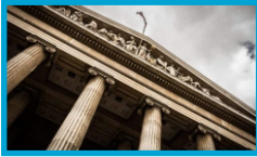
Building Repair and Maintenance
