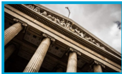
Building Repair and Maintenance
